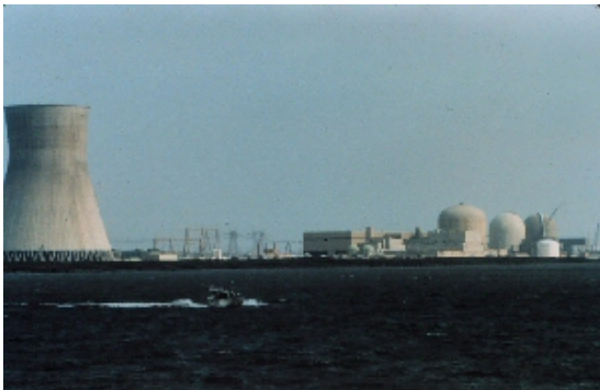
Nuclear power station
